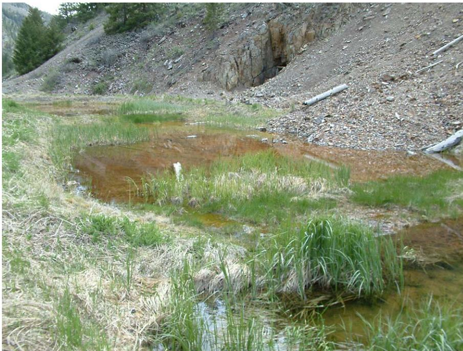
Fig. 2. Wetland treatment system for discharge from the King Solomon mine in Creede, CO.
